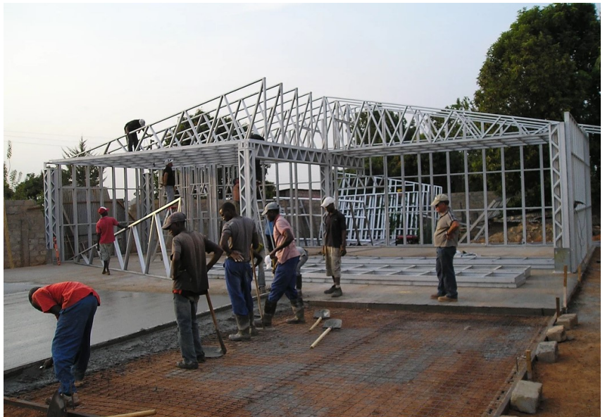
Steel Frame: Steel Home Company
