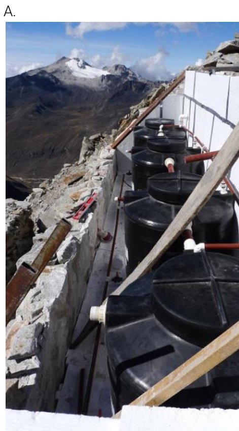
Figure 3 A. Implementation of rigid tank design in a high elevation location (Las Rocas Refuge 5130 masl). B. Tubular digester design including an insulated trench and greenhouse. Images borrowed from Dr. Jaime Martí-Herrero.
